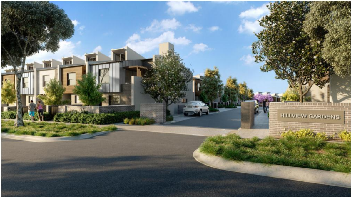
VIEW FROM HILLVIEW ROAD - ENTRY TO INTERNAL ROAD EAST
